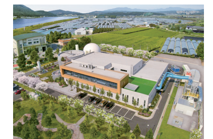
Chungju Foodwaste Bioenergy Center
